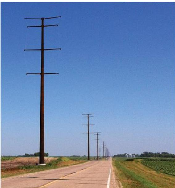
*Single pole steel structures will primarily be used to reduce land impacts; some locations may require two pole structures. Poles are between 140 and 170 feet tall and will be about 1,000 feet apart. Typically, a 150-foot wide right-of-way will be required.*
